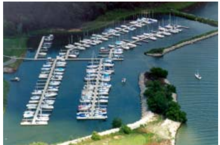
Boulder Access Marina as it appears today, with wide, stable concrete docks.
